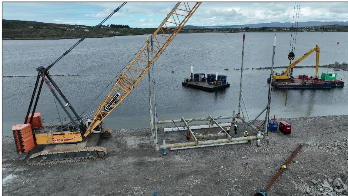
Figure 2-9: Bespoke frame used to accurately lower and position the foundation beams for the quay wall in the trench.
