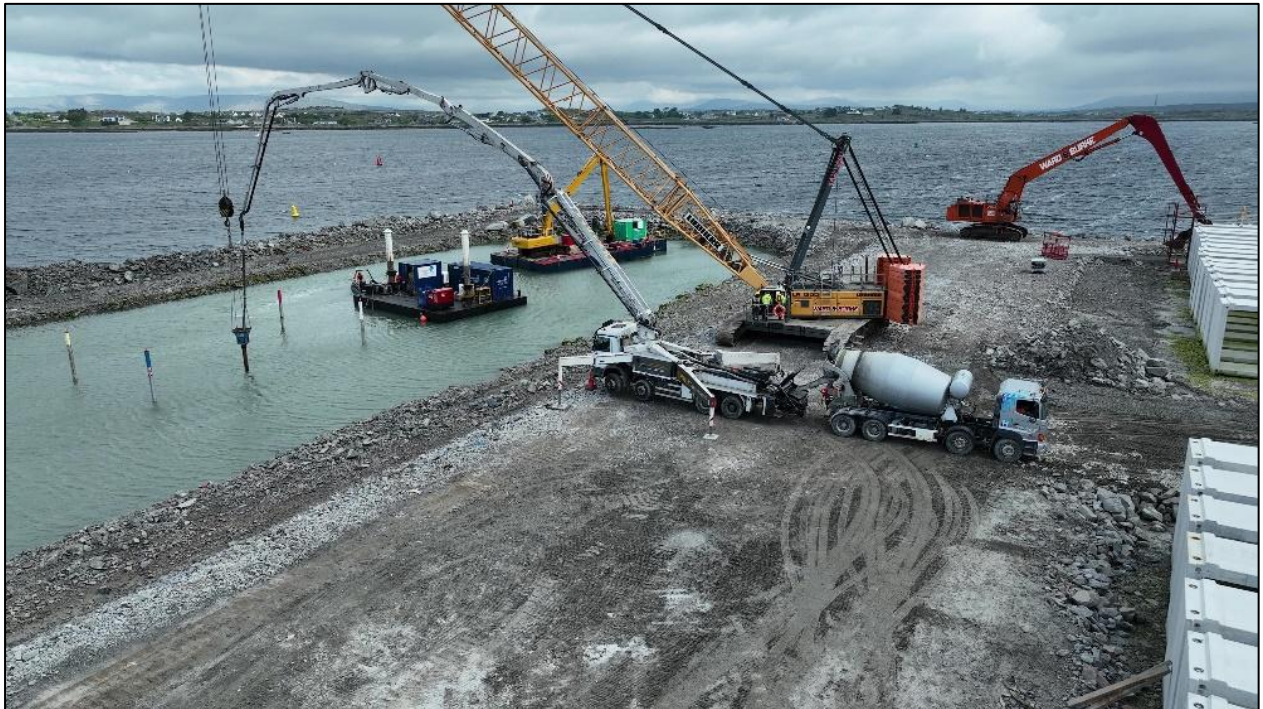
Figure 2-10: Liquid concrete being delivered via Tremie Pipe and directed by underwater divers to surround and hold the foundation beams in place.
