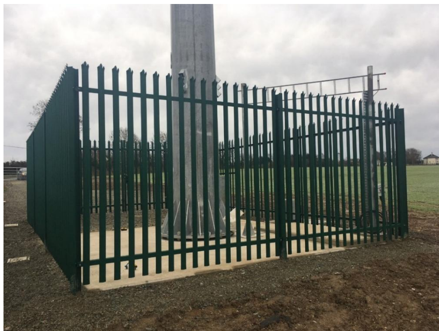
Figure 2-22 2.4m high Palisade Fencing
