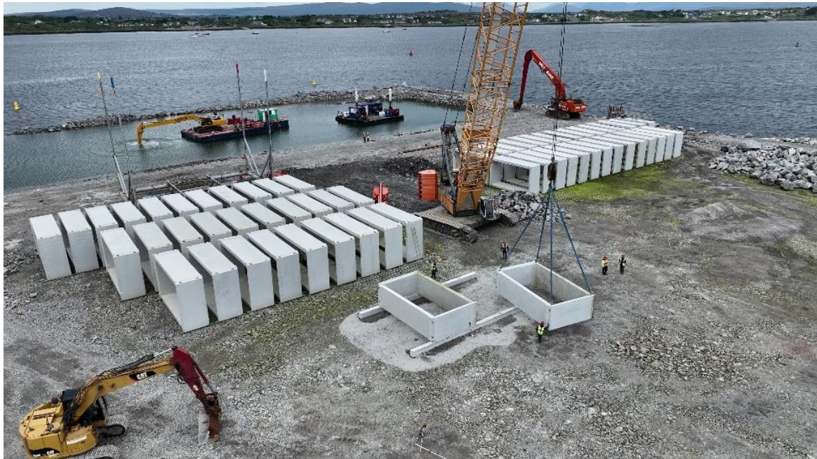
Figure 2-8: Photography of the (7m x 4mx 2m) concrete caisson boxes being positioned on precast concrete foundation beams positioned on the ground during a field trial on land.
