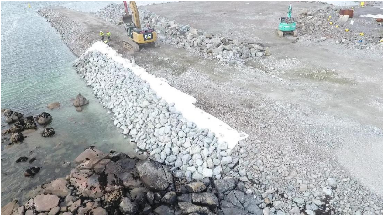
Figure 2-14: Construction of Rock Armour for the revetment (underlaid with geotextile).
