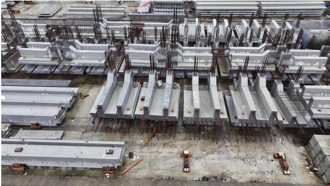
Figure 2-12: Precast wall sections to be placed on top of uppermost row of box caissons.
